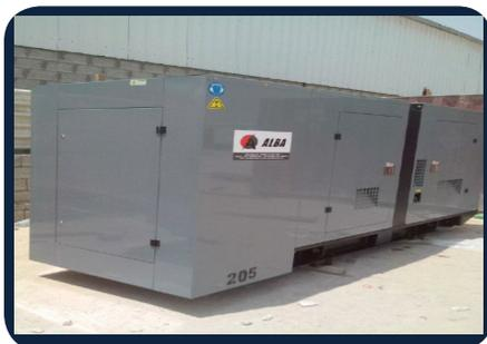
40 kva diesel generator set with sound attenuated canopy
