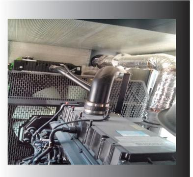
The roof and walls are insulated with rock wool and fibrous and metal protections. the whole exhaust line is covered by insulation iackets, insulated divider.
